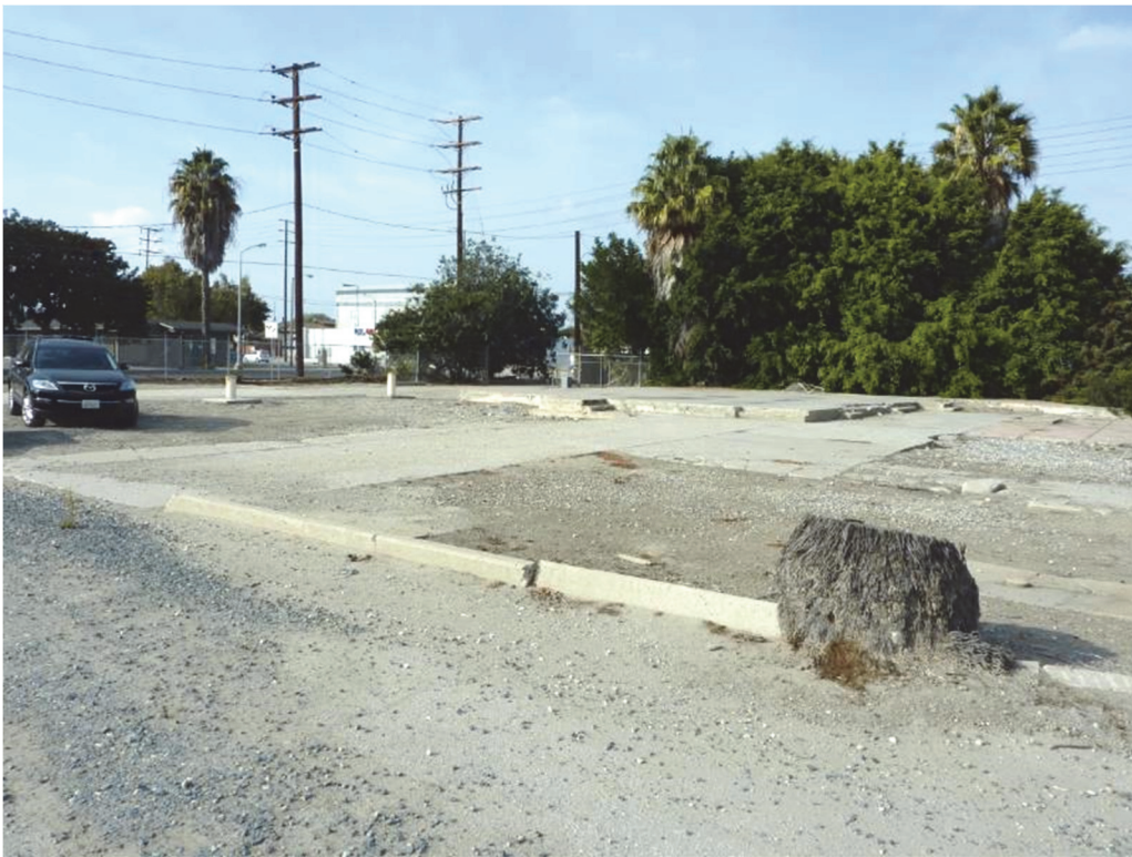
J-1. Looking to northwest in northwest corner of site over concrete foundation pads with groundwater monitoring wells in middle-distance left (11/18/2013).
