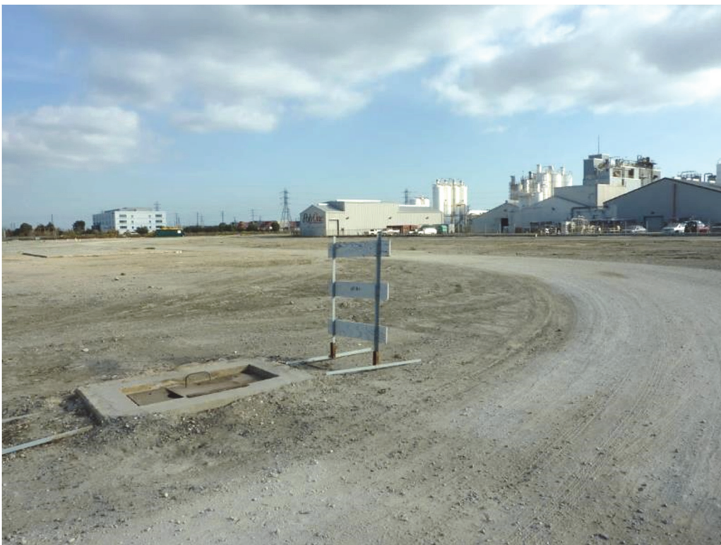
J-4. Sewer connection with PolyOne facility in background right and ARCO polypropylene building in background left (11/18/2013).
